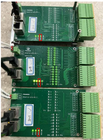
Fig. 11 EtherCAT communication established by IO board
